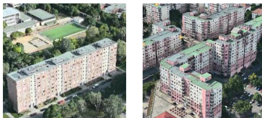
Figure 1. Prefabricated residential buildings with different geometric properties [9]
