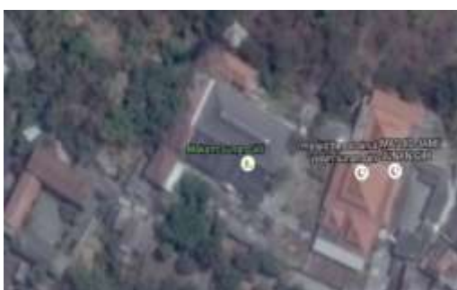
Fig. 10. Photo images AinalYaqien Mosque complex and SunanGiri Tomb complex built in the 15th century of SunanPrapen's rule
