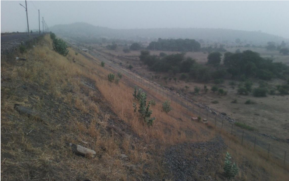
Figure 2: Downstream face of the dam
