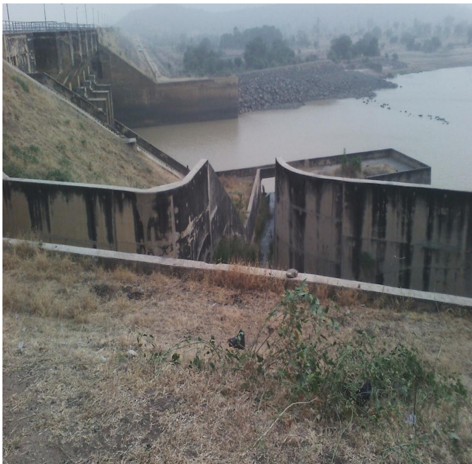
Plate 4: Spillway gate of Kiri Dam
