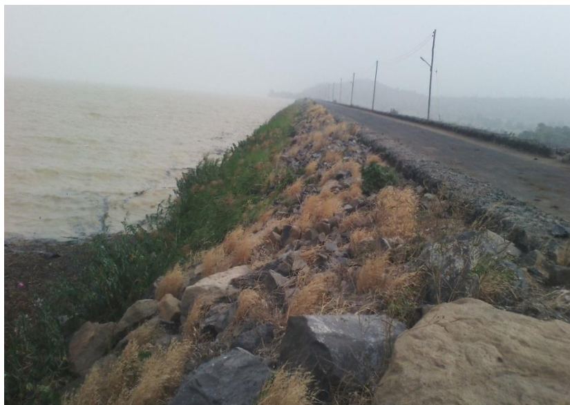
Figure 3: Upstream face of Kiri dam
