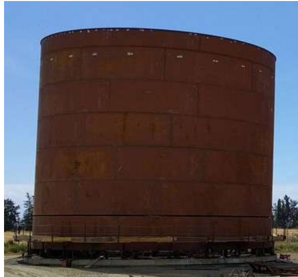
Figure1: Different shell courses in a cylindrical steel tank
