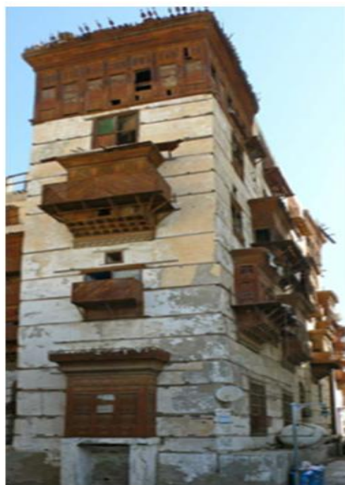
Figure 8: Jamjoom House, in Historic Jeddah.
