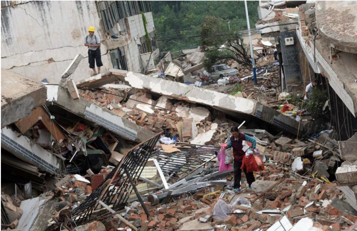
Figure 1.2 Disaster situation after earthquake in Ludian county
