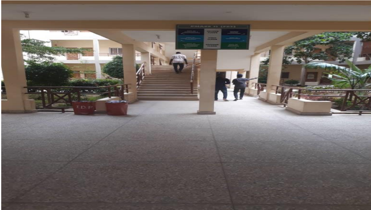
Plate VII: Staircase case with large circulation area, A.T.B.U Bauchi
