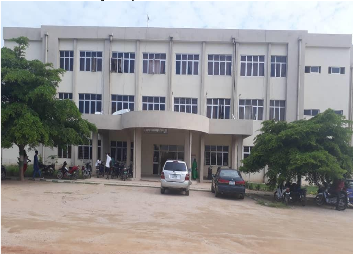
Plate II: Approach view to the main entrance of the faculty of environmental technology, A.T.B.U Bauchi Source: Researcher Field Work(2022)
