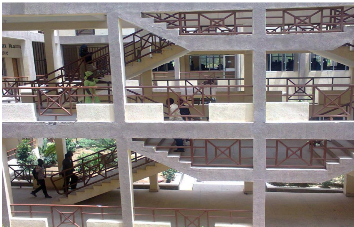
Plate V: Central staircase for vertical circulation of faculty of environmental technology A.T.B.U Source: Researcher Field Work, (2018)
