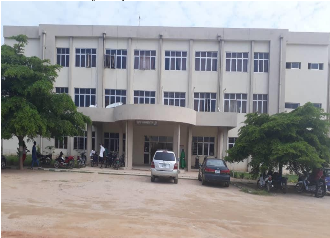
Plate II: Approach view to the main entrance of the faculty of environmental technology, A.T.B.U Bauchi
