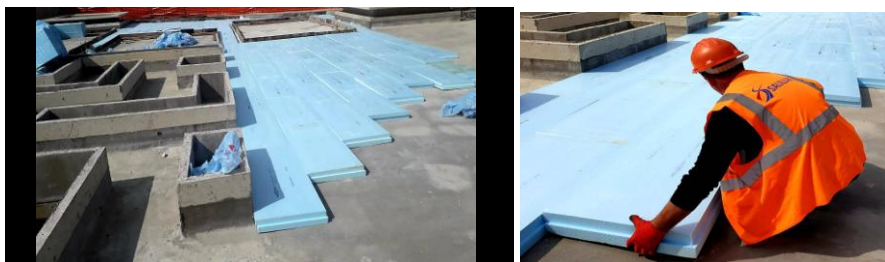
Figure 5. XPS implementation;source: Izoterm Albania [5]
