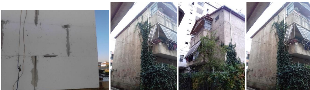
Figure 6.VillaFeritRragami during the application of EPS and the current situation; Luca Ndertim[6]
