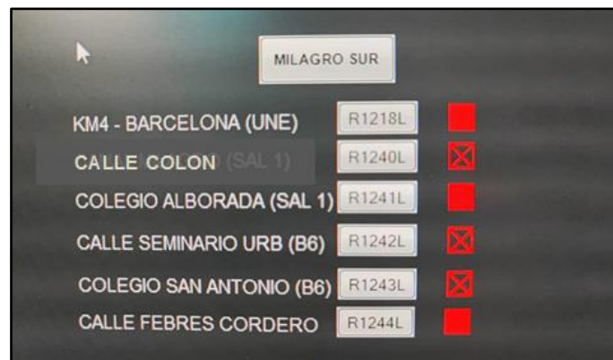
Figure 2: Monitoring of faults in real time in the SCADA system.
