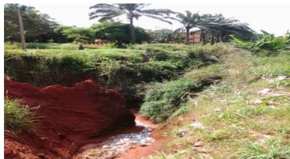
Fig 1: A picture of gully at Uruegbe in Umuoji
