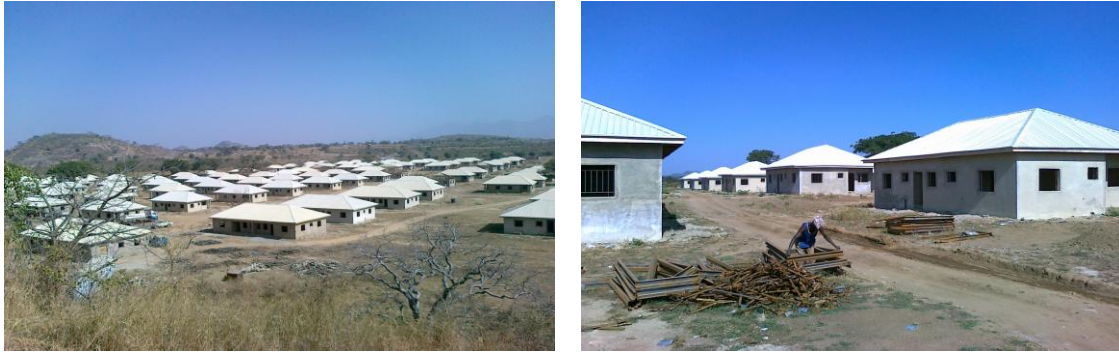
PLATE 1. Dungal Housing Estate under Construction.
