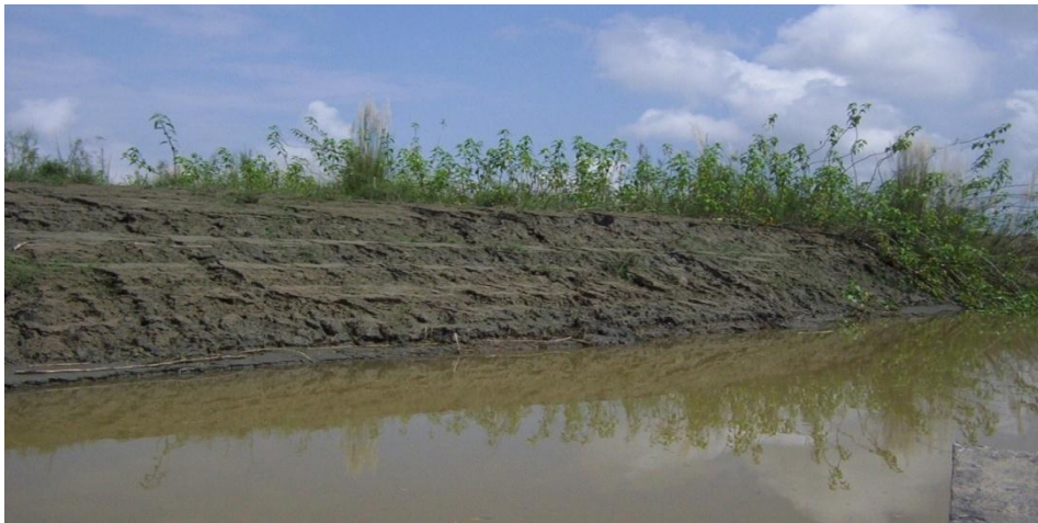
Photo- 2: Water level marks in the Brahmaputra river bank.
