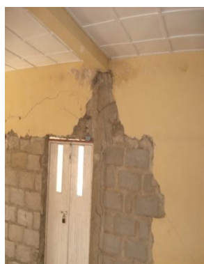
plate iv: Re-constructed column & wall
