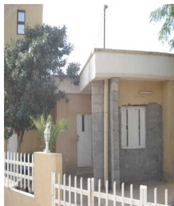
Plate ii: Re-constructed portion of wall
