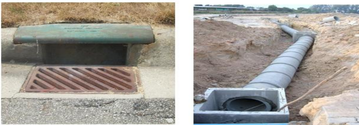
Figure 5 Collector of surface water
