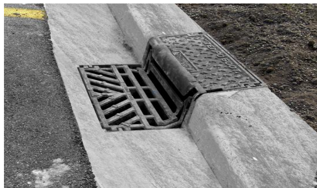
Figure 8 Hinged Kerb Gully gate
