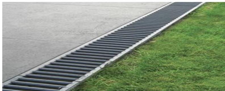
Figure 11 Linear Drainage System
